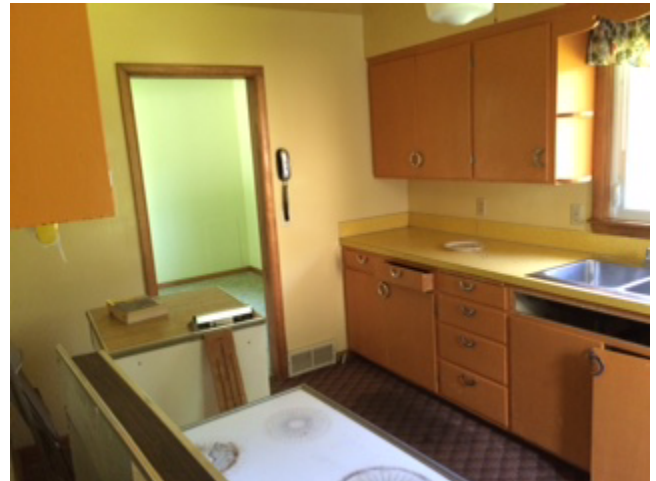
NW View into Kitchen from Breezeway Entry
