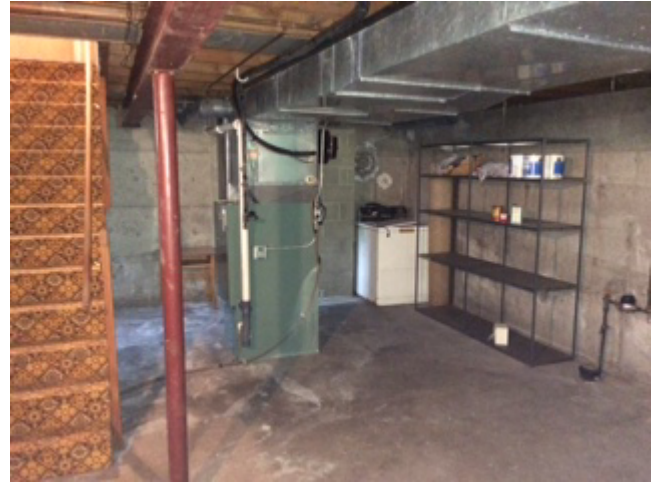
SE View in Basement
