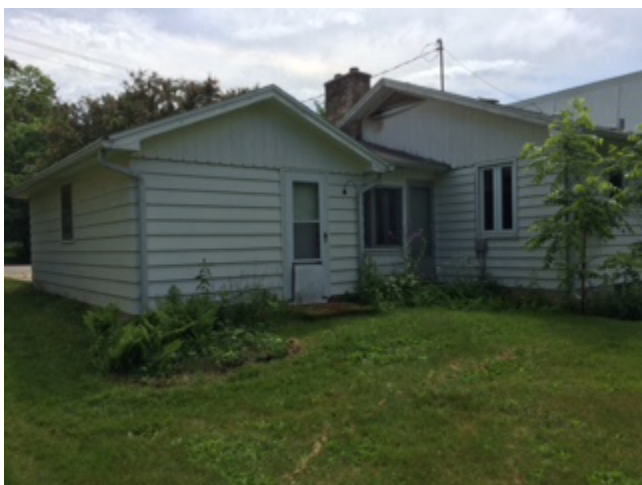
SW View of North Elevation
