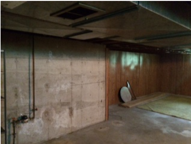
SW View in Basement
